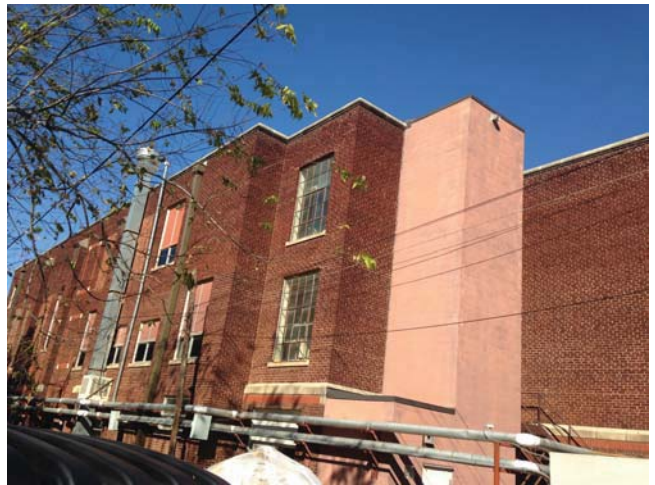
Movement at elevator—new windows
