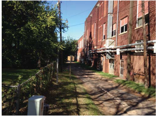
Clean up exterior utilities/ alley access
