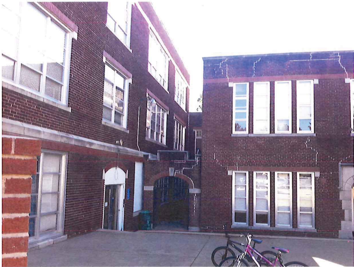
Picture #11 – Repointed Mortar Joints
