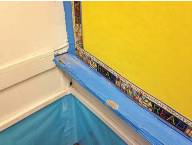
Termite Damage
