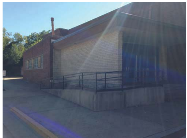
Gym exterior in better condition
